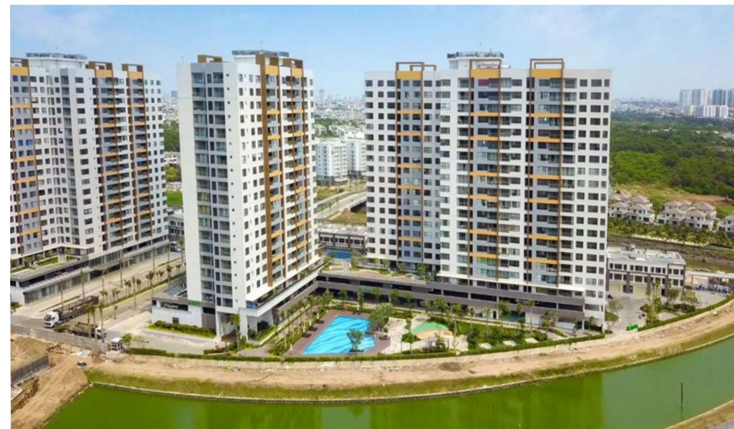
Mizuki construction progress December/2019
