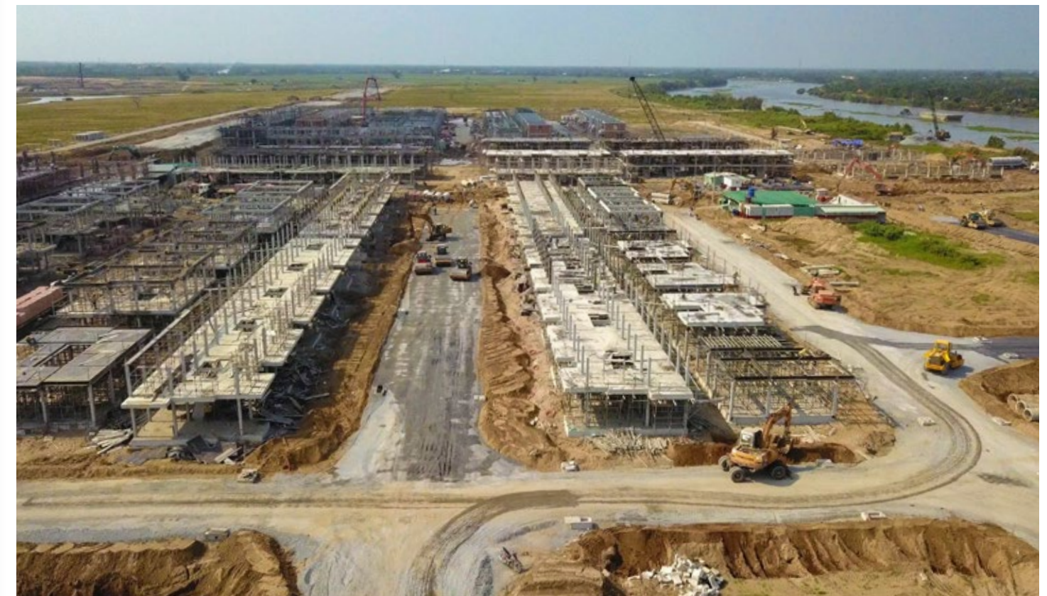
Waterpoint construction progress December/2019
