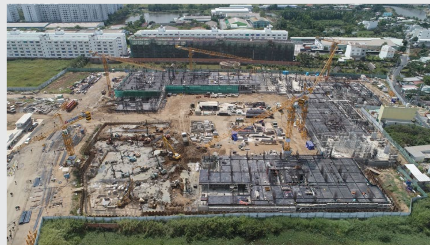
Akari City construction progress December/2019
